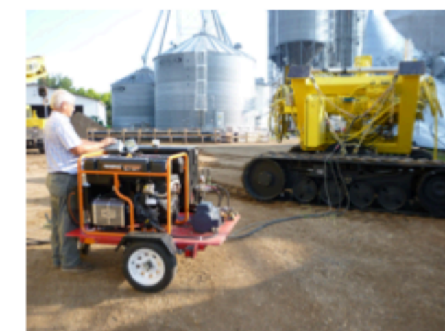
Moving Tracks and PWR Plant with HydroPac
