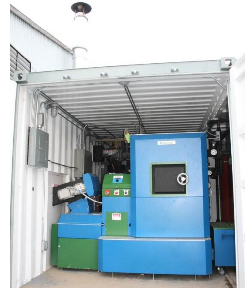
ACT Bioenergy Wood Boiler
