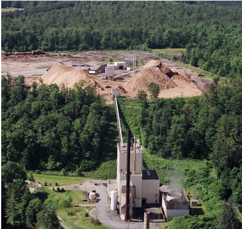
Lyonsdale Biomass Power Plant, Lyons Falls, NY Photo: Catalyst Renewables
